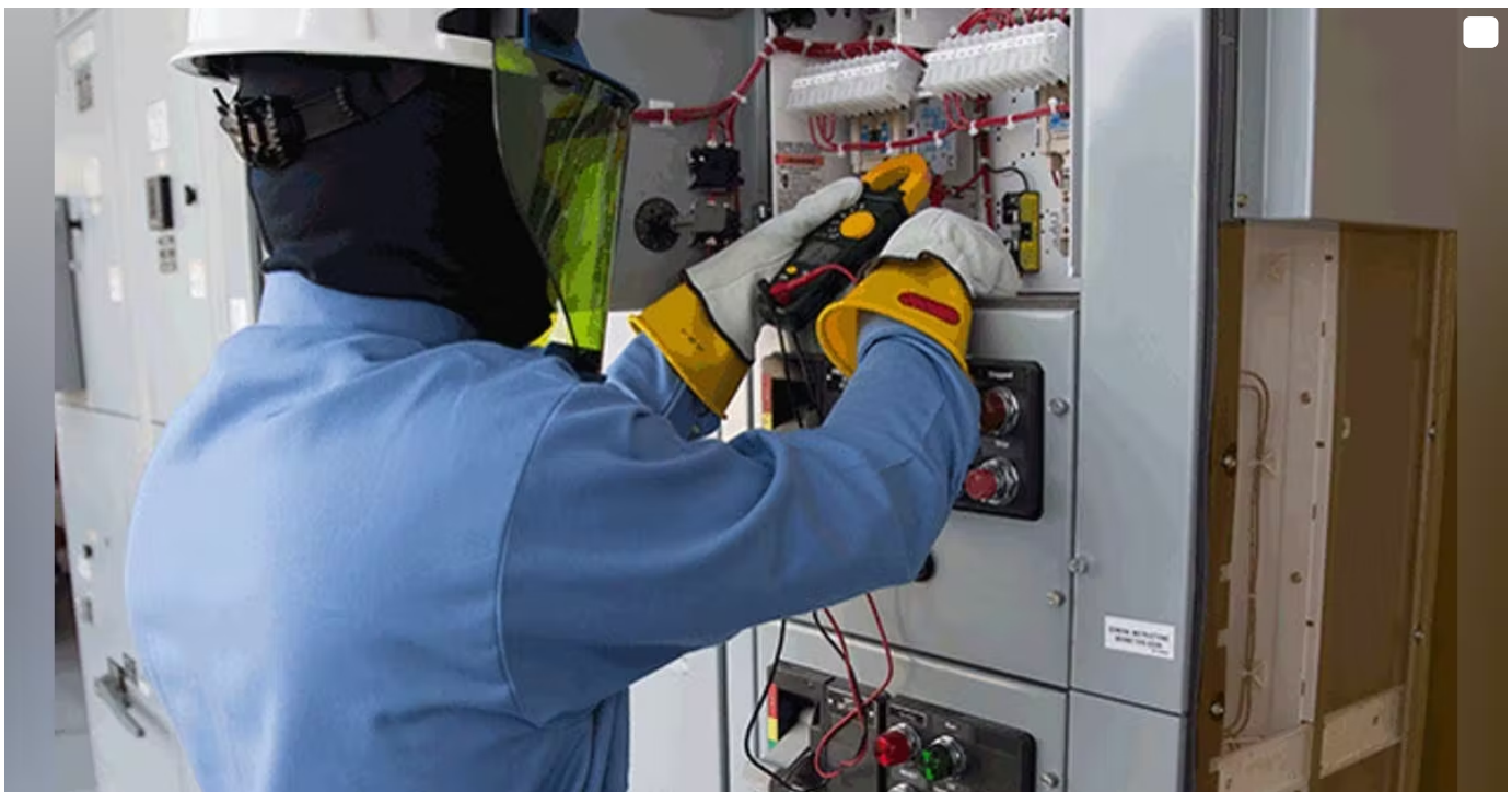
An electrical worker is geared up in arc flash workwear, which includes rubber insulated safety gloves, a hard hat, and face shield.
